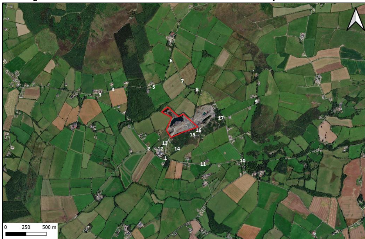
Figure 15.5: Locations from which the visual assessment of the subject site was made
